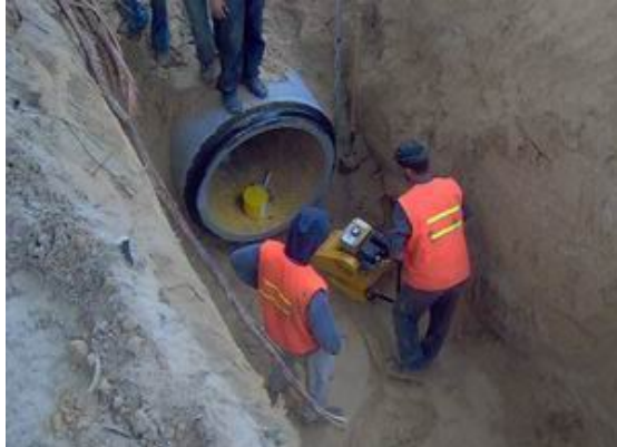
Installing the Main Inlet Pressure Line (Completed)
