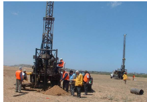
Geotechnical Investigations in KY WWTP Eastern (Completed)
