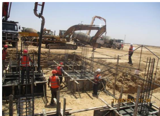
Casting Reinforced Concrete for Admin Building and Plain Concrete for Aeration Tank on 17 May 2017
