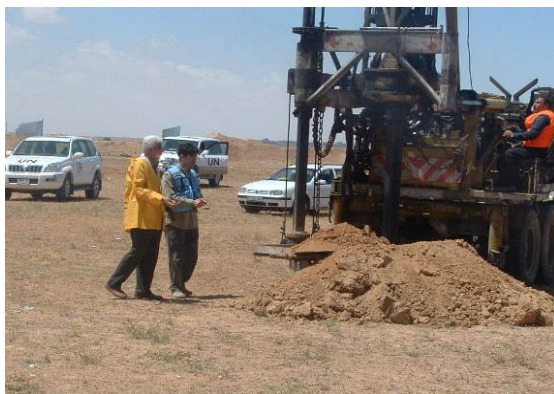
Geotechnical Investigations in KY WWTP Eastern (Completed)
