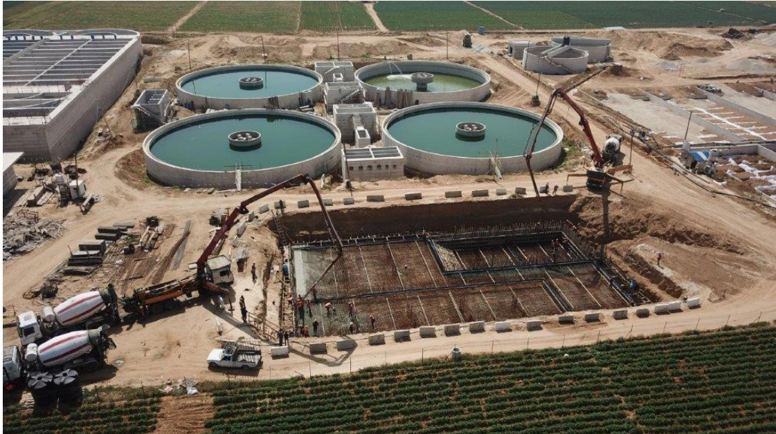
Steel Reinforcement and casting Concrete for the Sand Filter in March 2018
