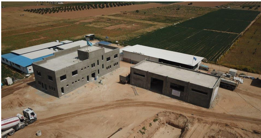
Executed Works for the Admin Building and Workshop in March 2018
