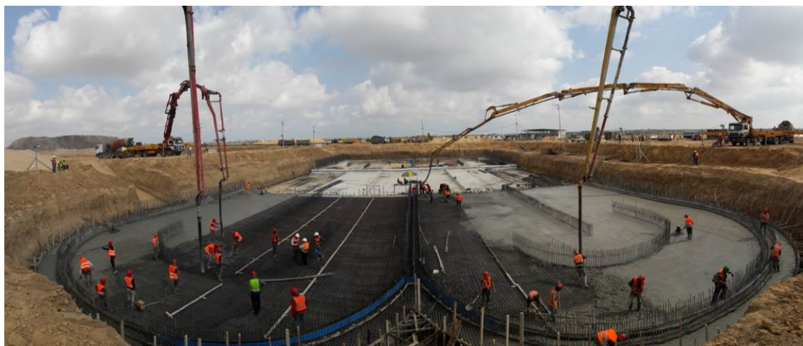
Casting Reinforced Concrete for the Foundation of the Aeration Tank on 20 June 2017
