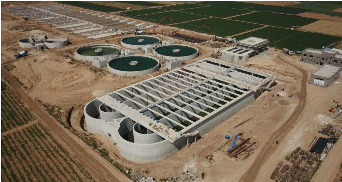
Casted Reinforced Concrete for the Aeration Tank in March 2018
