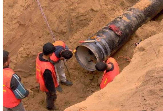
Installing the Main Inlet Pressure Line (Completed)
