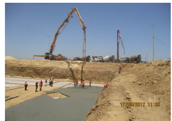
Casting Reinforced Concrete for Admin Building and Plain Concrete for Aeration Tank on 17 May 2017
