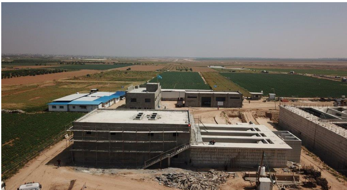
Casted Reinforced Concrete for the Pre-Treatment Building in March 2018
